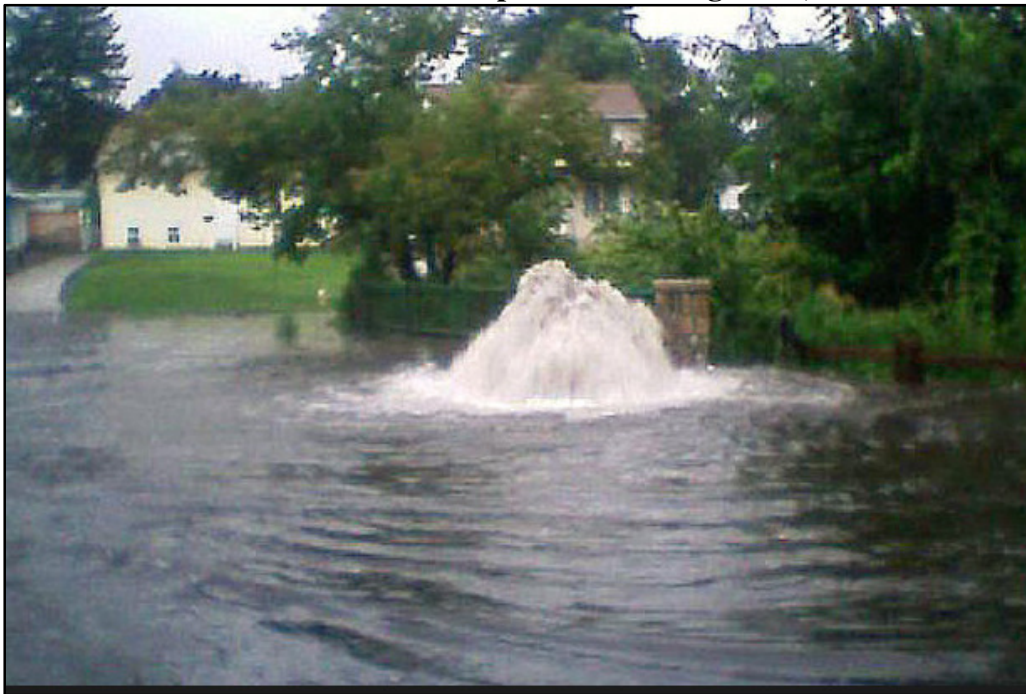
Photo 4.4-2: Dickinson Siphon SSO – August 28, 2012
