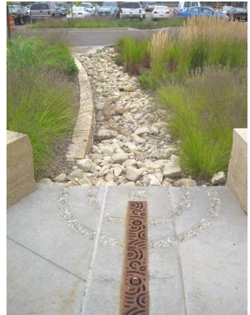
Drain collects runoff from impervious surface and directs it to rain gardens in Saint Paul, MN.
