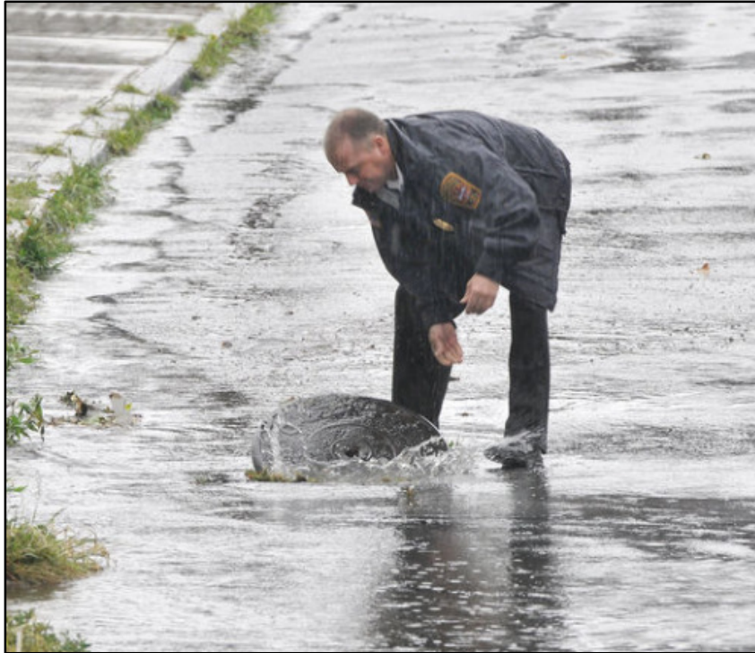
Photo 4.4-1: Dickinson Siphon SSO – August 28, 2012
