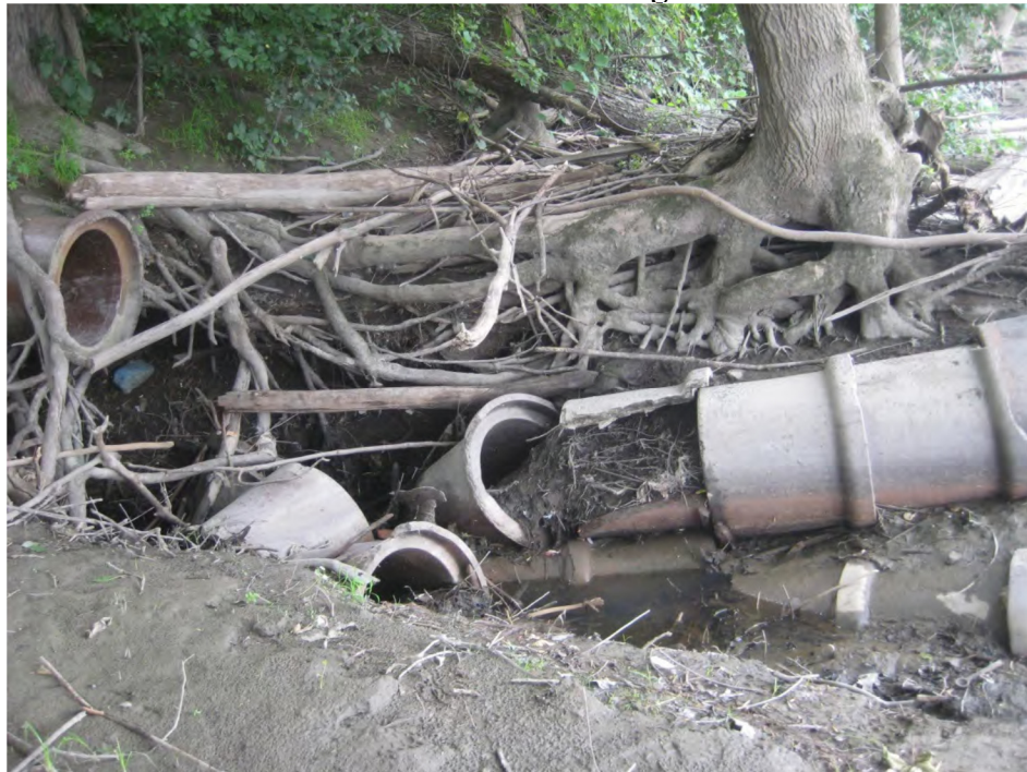
Photo 4.4-3: CSO 018 Existing Condition
